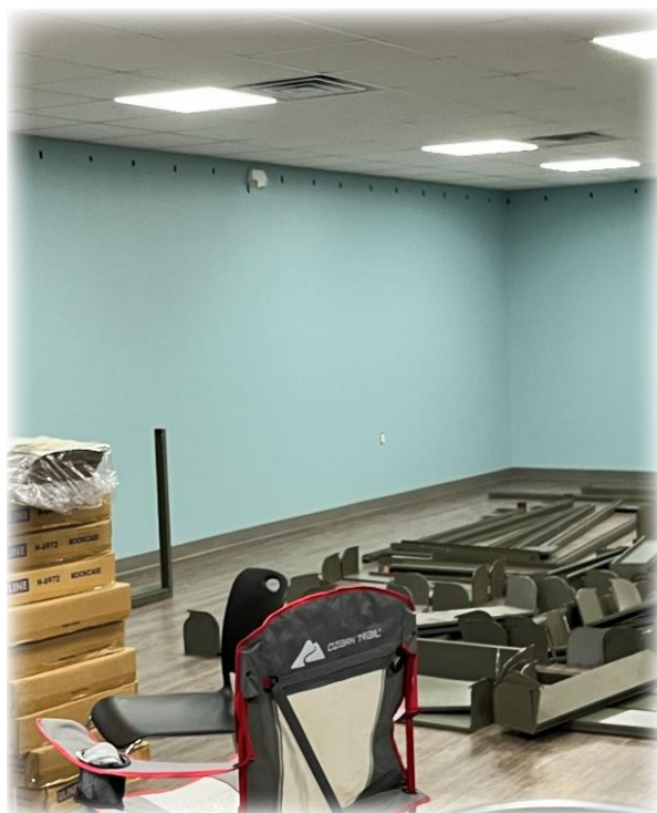
Painting in progress. The director and her husband spent Labor Day Weekend 2025 disassembling shelving, loading it on a trailer, moving, unloading, reassembling, and rebuilding it in the new space.
